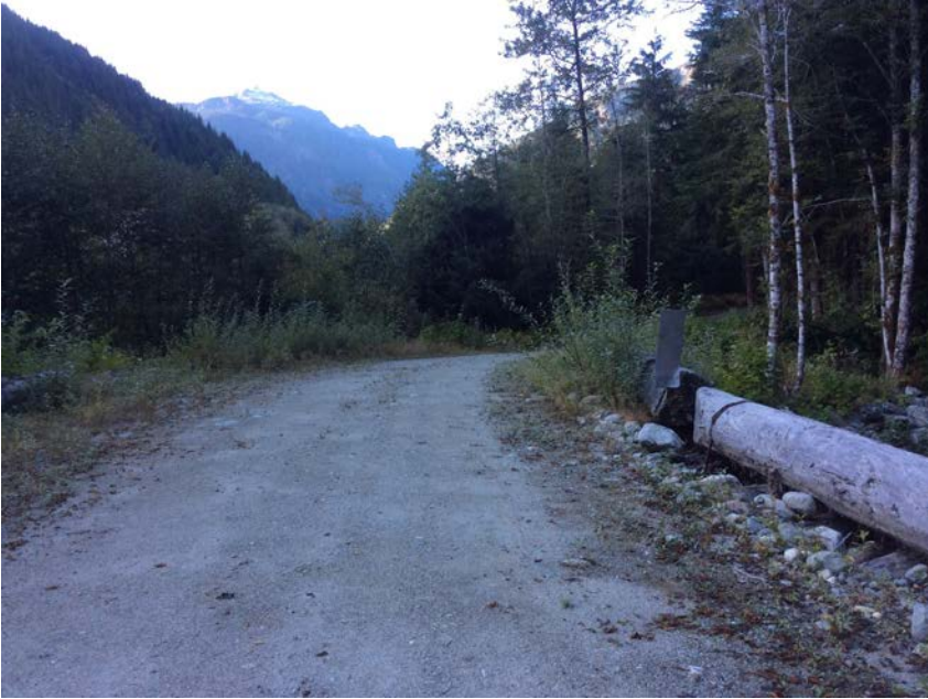
Right approach viewed from bridge
