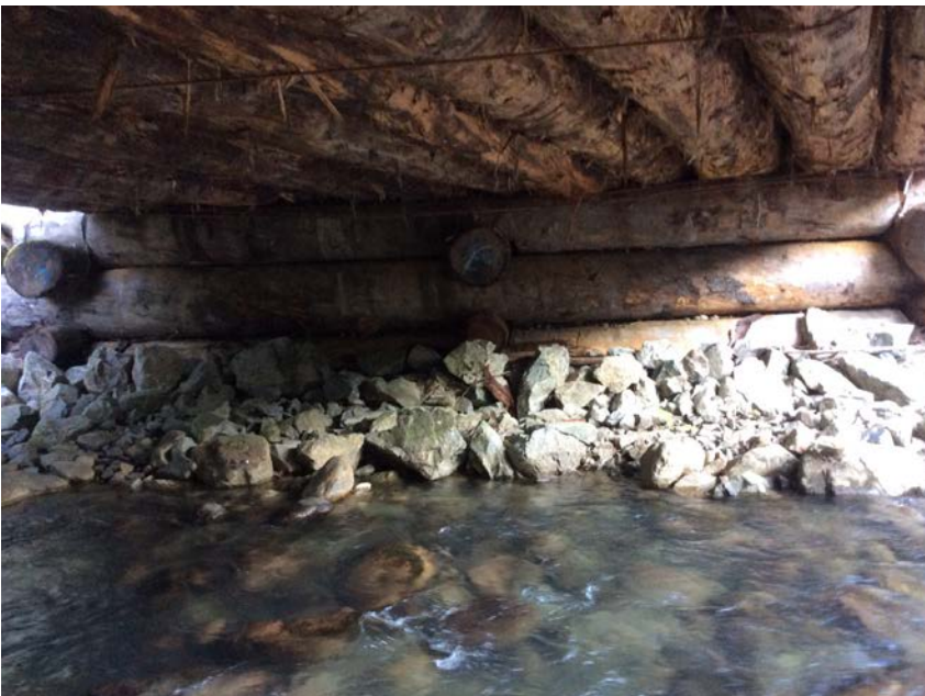
Left Bank Abutment when facing downstream
