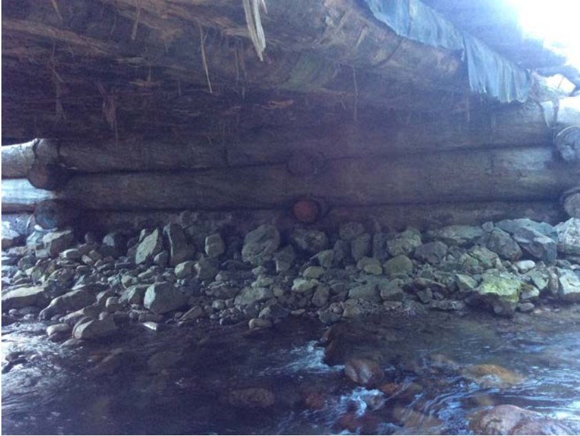
Right Bank Abutment when facing downstream
