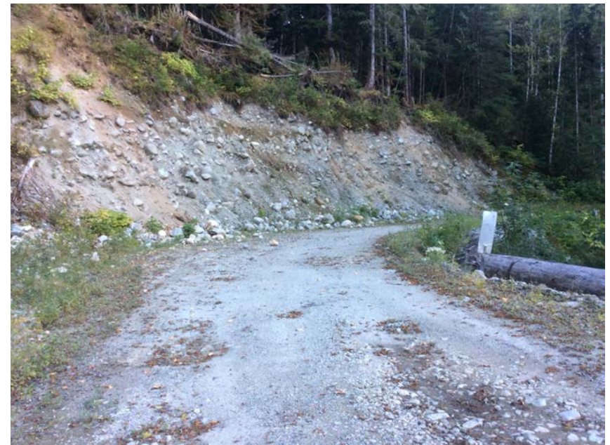
Left approach viewed from bridge
